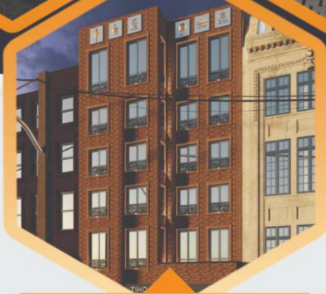
Smart system Avand commercial treatment building
