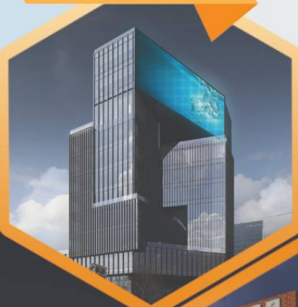
Smoke control system Mika-Knots Tower
